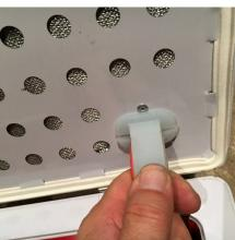
c. Minimize gapping and ensure the upper and lower lip of the wire way is properly seated on outside of box lid.
